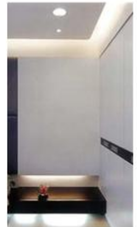
4. Lighting. Lighting to be concealed where possible. All lighting to be dimmable. Light sources to be concealed within "light shelves" to soffit and down lighters within furnishings recessed ceiling areas.
