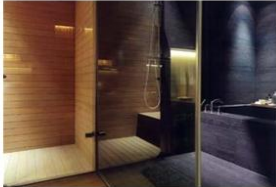
1. Shower Enclosure. The shower areas are custom finished areas, with slate panelling to the walls, frameless glass openings, concealed shower tray, with teak shower grate.
