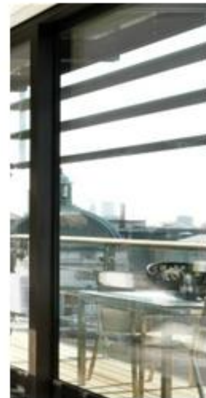
5. Windows/Frames. All windows to be low-E toughened DGUs with minor solar tints. All window frames to be powder coated (Grey/Black) Aluminium. Mullions to be deep section. Heating to be under floor with additional heating/cooling ventilation grills adjacent to window apertures.
